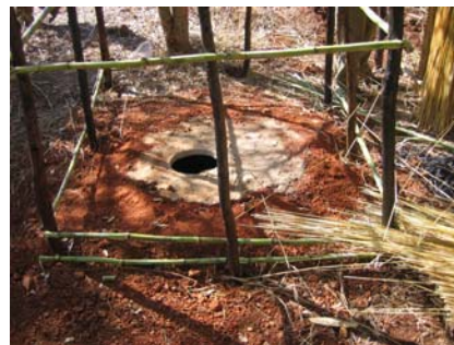
Figure 3-50: Gum poles, reeds and grass used to build the wall
