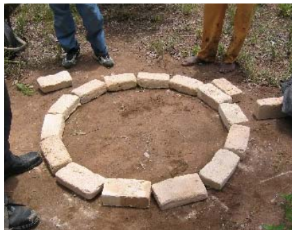
Figure 3-5: Ring of bricks for the mould
