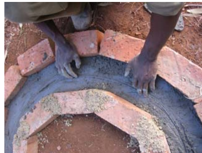
Figure 3-44: Addition of wire for reinforcement
