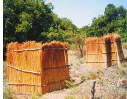
Figure 3-38: Toilet houses without a roof
