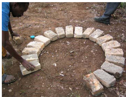
Figure 3-10: Forming the brick ring beam
