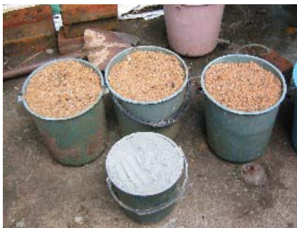
Figure 3-7: Measuring cement and river sand
