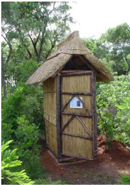
Figure 3-1: Simple compost toilet built on rectangular slab
