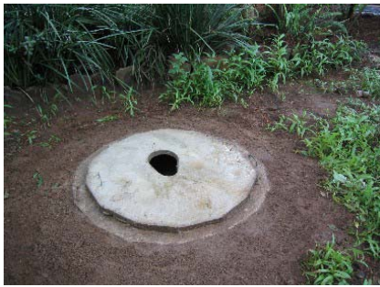
Figure 3-20: Toilet slab placed on ring beam
