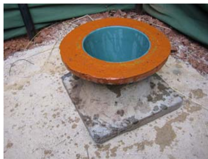
Figure 3-52: Low-cost pedestal on top of slab
