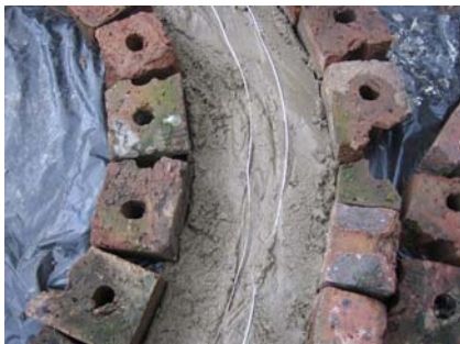
Figure 3-31: Wire reinforcement added
