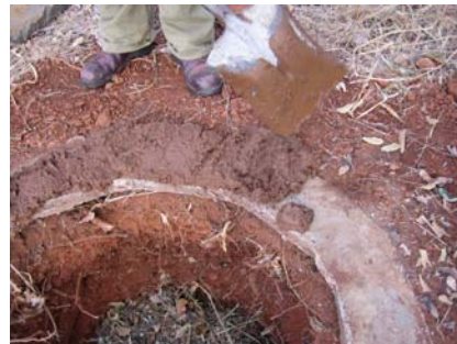
Figure 3-48: Anthill mortar packed around ring beam
