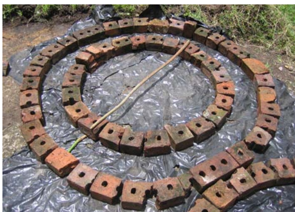
Figure 3-28: Two brick circles for ring beam mould
