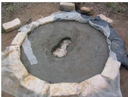
Figure 3-9: Mould after removal of squat hole insert
