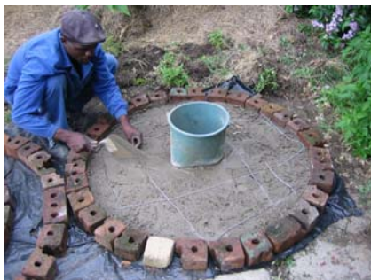
Figure 3-26: Wires added for reinforcement
