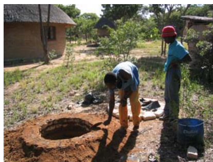
Figure 3-34: Packing soil around the brick ring beam
