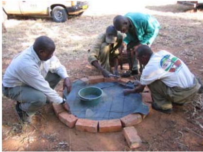
Figure 3-41: Laying down reinforcement wires
