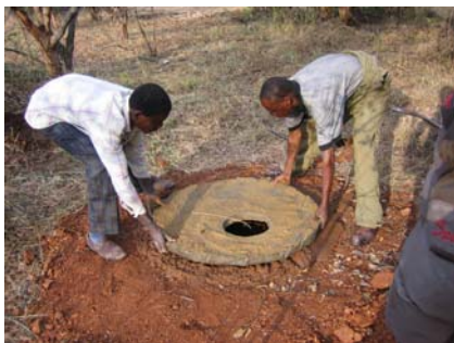
Figure 3-49: Slab placed over ring beam
