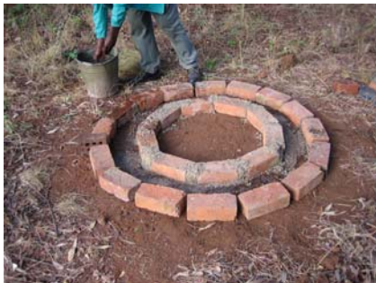
Figure 3-43: Ring beam mould using bricks
