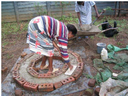
Figure 3-16: Levelling off the concrete
