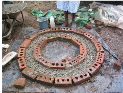
Figure 3-15: Cement and wire reinforcement added to mould
