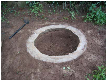
Figure 3-18: Digging of hole inside ring beam
