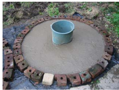
Figure 3-27: Remainder of concrete mix added and levelled-off
