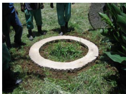
Figure 3-35: Placement of the concrete ring beam
