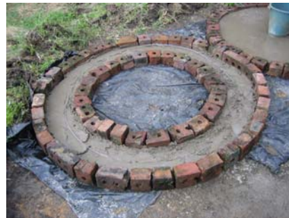
Figure 3-30: Concrete mix added to mould
