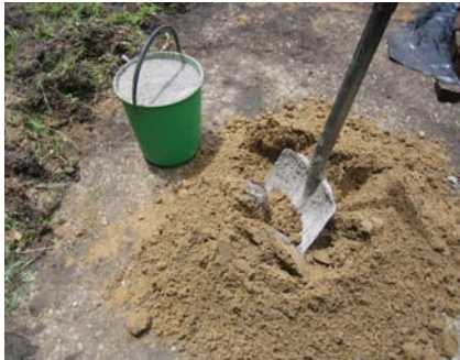
Figure 3-24: Mixing the cement and river sand
