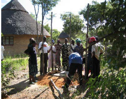
Figure 3-37: Using poles to build the toilet house
