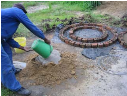
Figure 3-29: Mixing the cement and river sand
