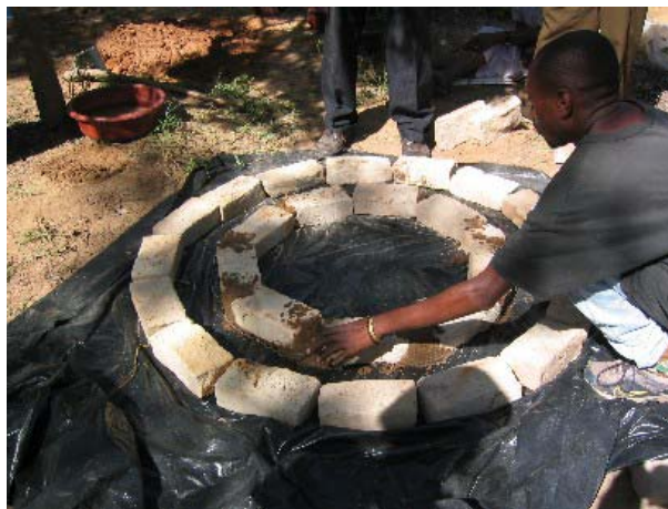
Figure 3-13: Brick mould on top of plastic sheet
