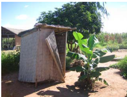
Figure 3-39: Toilet house built with local materials
