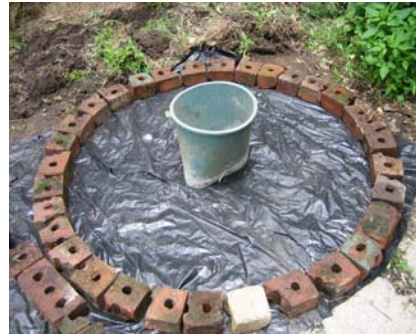
Figure 3-23: Shaped bucket to make the squat hole
