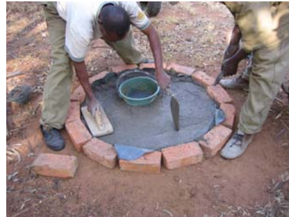
Figure 3-42: Levelling-off the concrete mix
