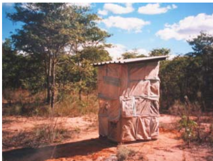
Figure 3-57: A portable structure built using a frame of poles
