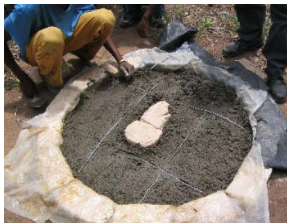
Figure 3-8: Cement and reinforcing wires in mould
