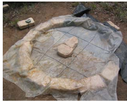
Figure 3-6: Sheet of plastic laid in the mould
