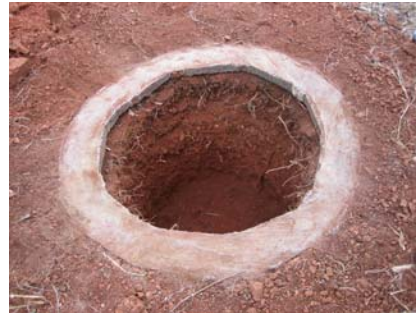
Figure 3-46: Pit dug inside ring beam
