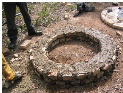
Figure 3-12: Completed brick ring beam
