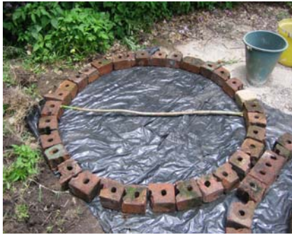
Figure 3-22: Circle of bricks 1.15m in diameter
