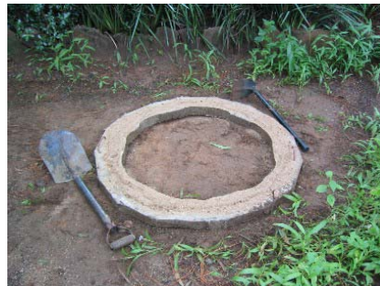
Figure 3-17: Completed ring beam
