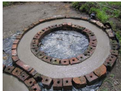
Figure 3-32: Remainder of concrete mix added and levelled-off
