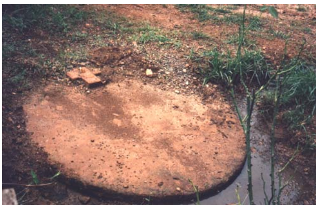
Plate 4.30. Photos from the same house showing sullage not properly connected to the pit
