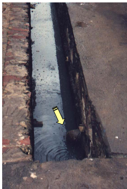
Plate 4.12. Discharge of excreta into the drainage channel
