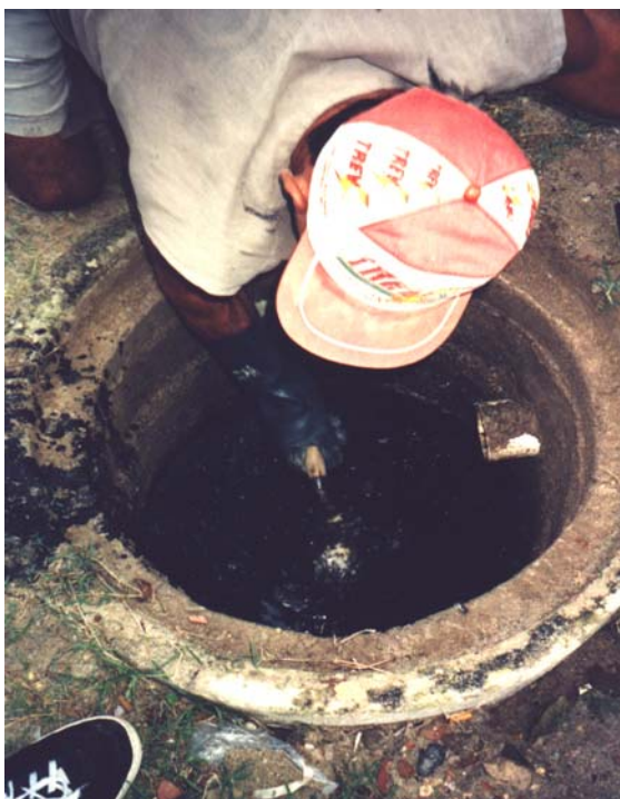
Plate 4.63. Removal of sand
