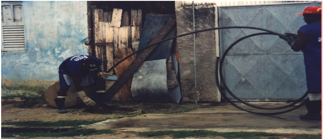
Plate 4.61. Workers using the hose to unclog the pipeline
