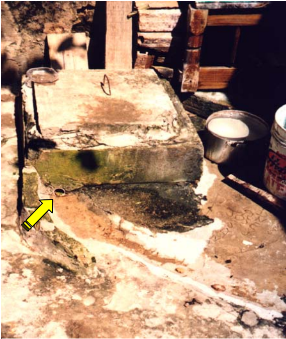
Plate 4.31. Entry hole for the discharge of stormwater into the inspection chamber.
