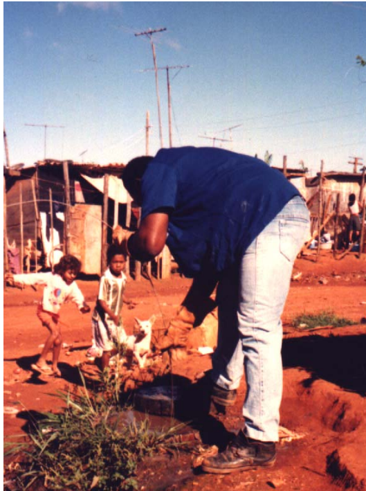
Plate 4.43. A member of the maintenance crew using a steel cable to displace clogging material
