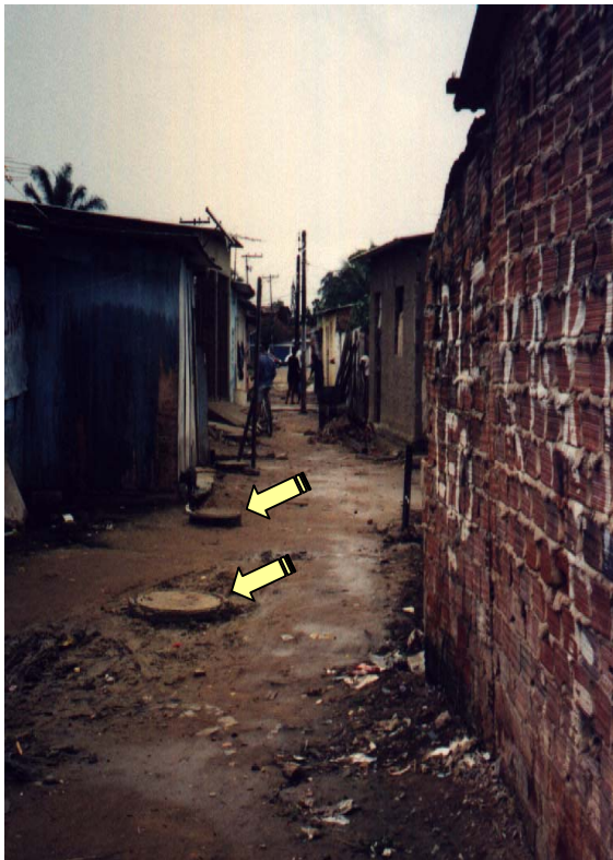
Plate 4.54. Favela of Campo do Piolho – the arrows show the inspection chambers of condominal sewer.
