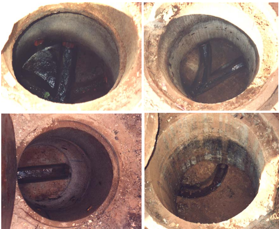
Plate 4.47. Different shapes of the bottom of inspection chambers.
