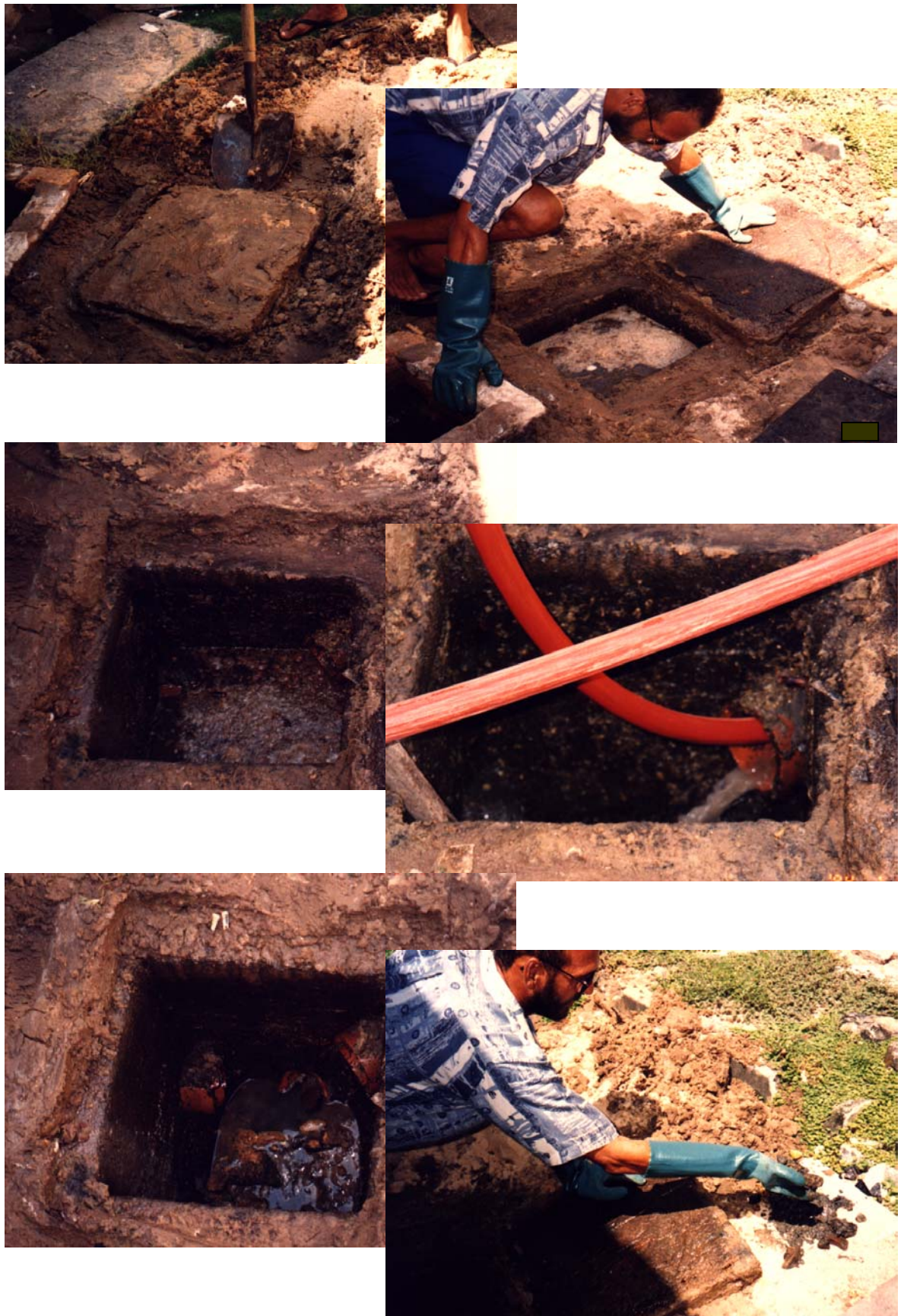
Plate 4.35. Cleaning out another condominial sewer – this time the cause of the problem was solid waste and stones inside the sewer.
