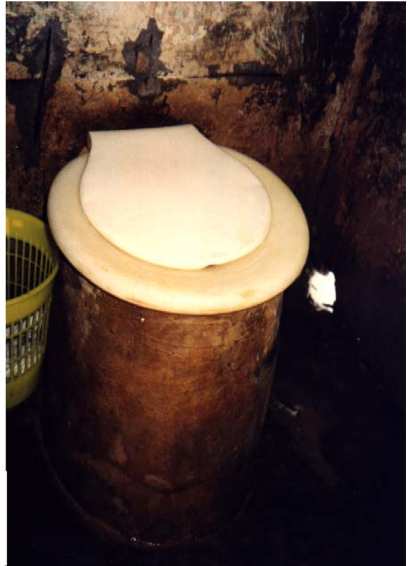
Plate 4.2. Pre-cast concrete riser to secure the toilet bowl
