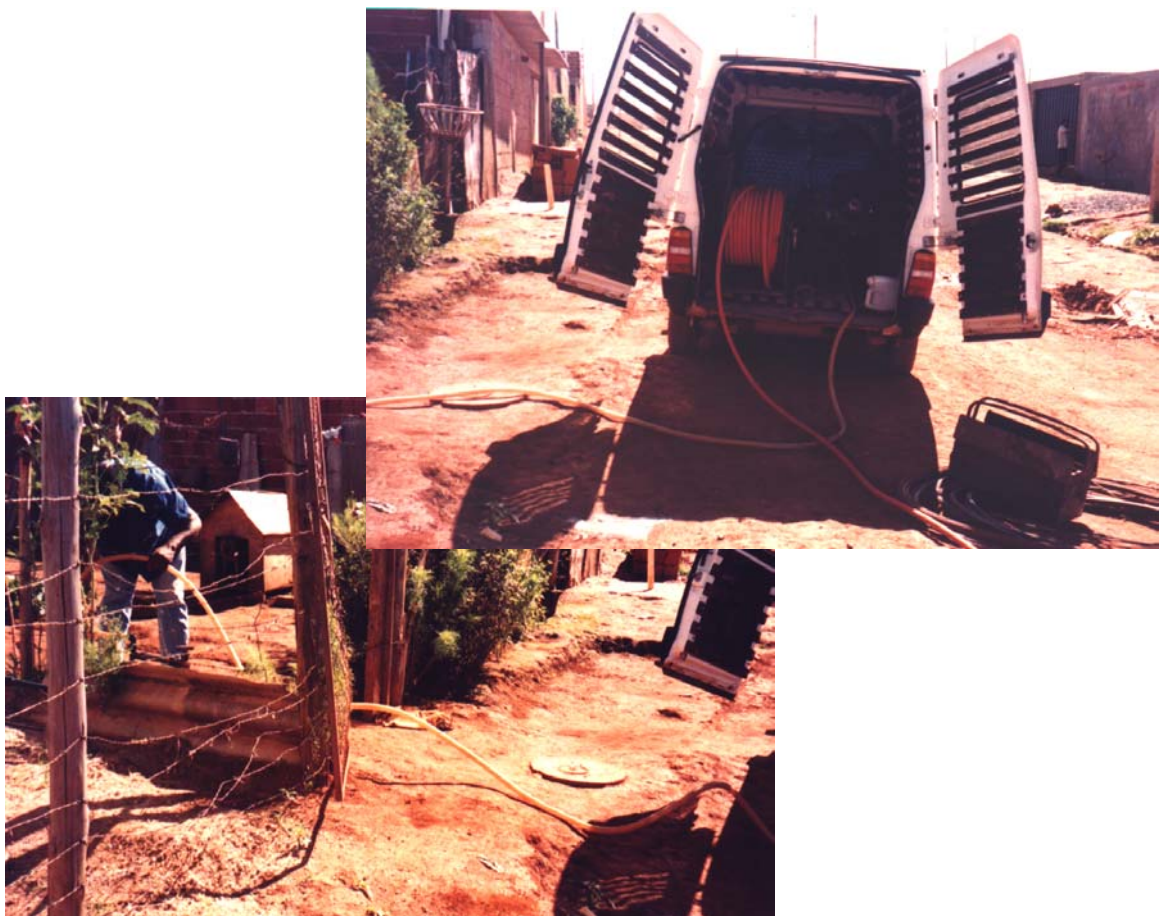
Plate 4.45. The water jet equipment being connected to a user's tap
