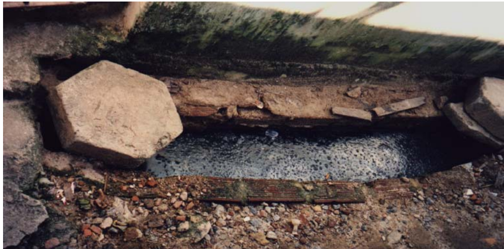
Plate 4.56. Section of a drainage channel in the Sigismundo favela.
