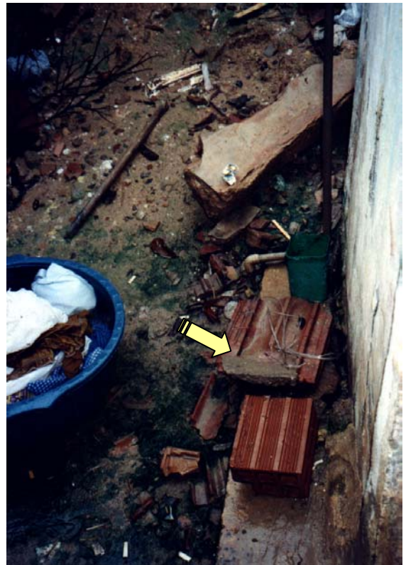
Plate 4.16. Brick covering the vent-pipe hole.
