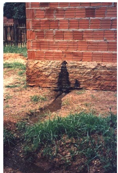
Plate 4.30. Photos from the same house showing sullage not properly connected to the pit
