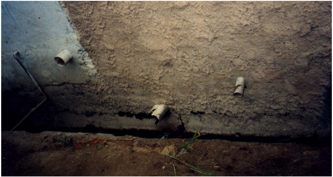
Plate 4.53. Household wastewater being discharged into drainage channels
