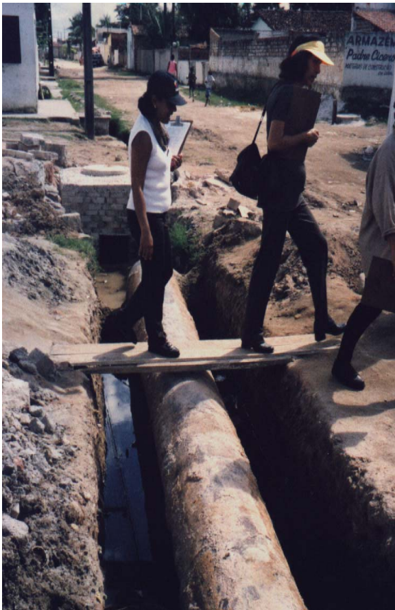
Plate 4.51. Drainage construction taking place in the Mangueira area
