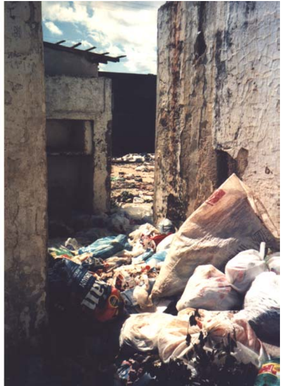
Plate 4.8. Interior of the composting unit.
