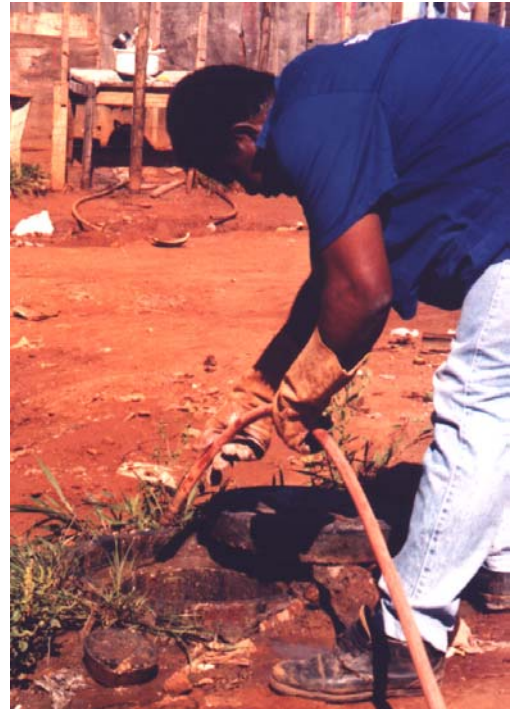
Plate 4.44. The utilisation of the water jet to clear clogging material
