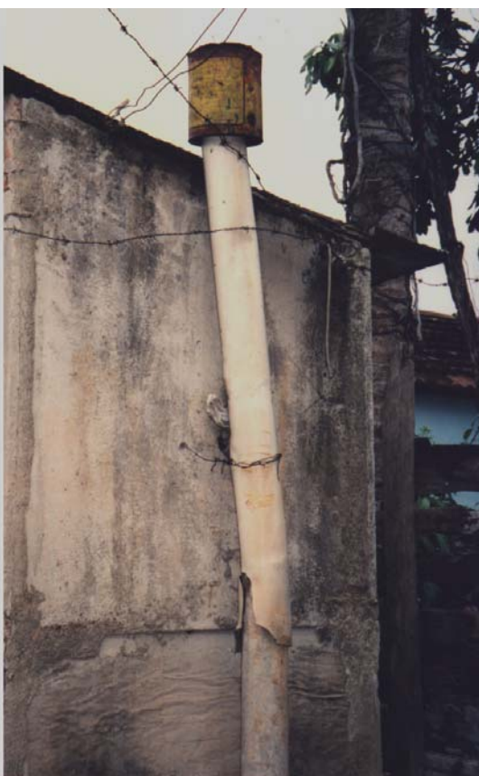
Plates 4.13. and 4.14. Details of a vent-pipe found with one of the latrines – note the tin blocking the vent-pipe and the positioning of the pipe.
