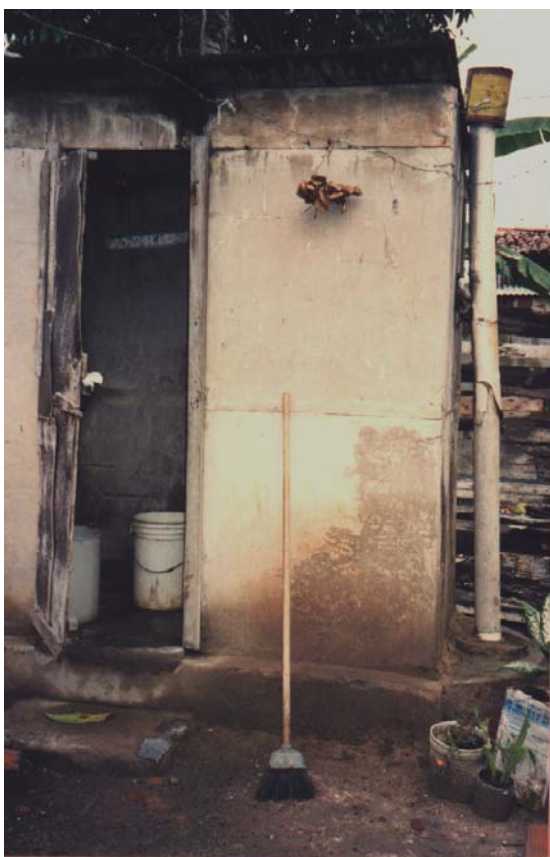
Plates 4.13. and 4.14. Details of a vent-pipe found with one of the latrines – note the tin blocking the vent-pipe and the positioning of the pipe.
