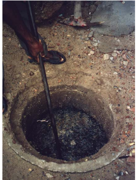
Plate 4.60. Close up of one of the inspection chamber
