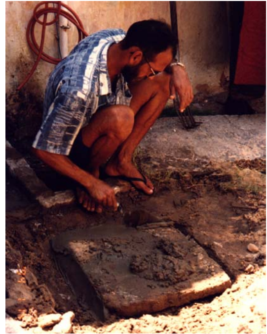
Plate 4.32. A CAERN crew member re-sealing the inspection chamber cover after a maintenance service.
