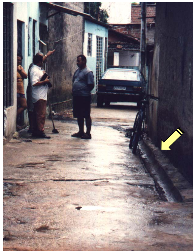
Plate 4.3. Channel for microdrainage and sullage collection
