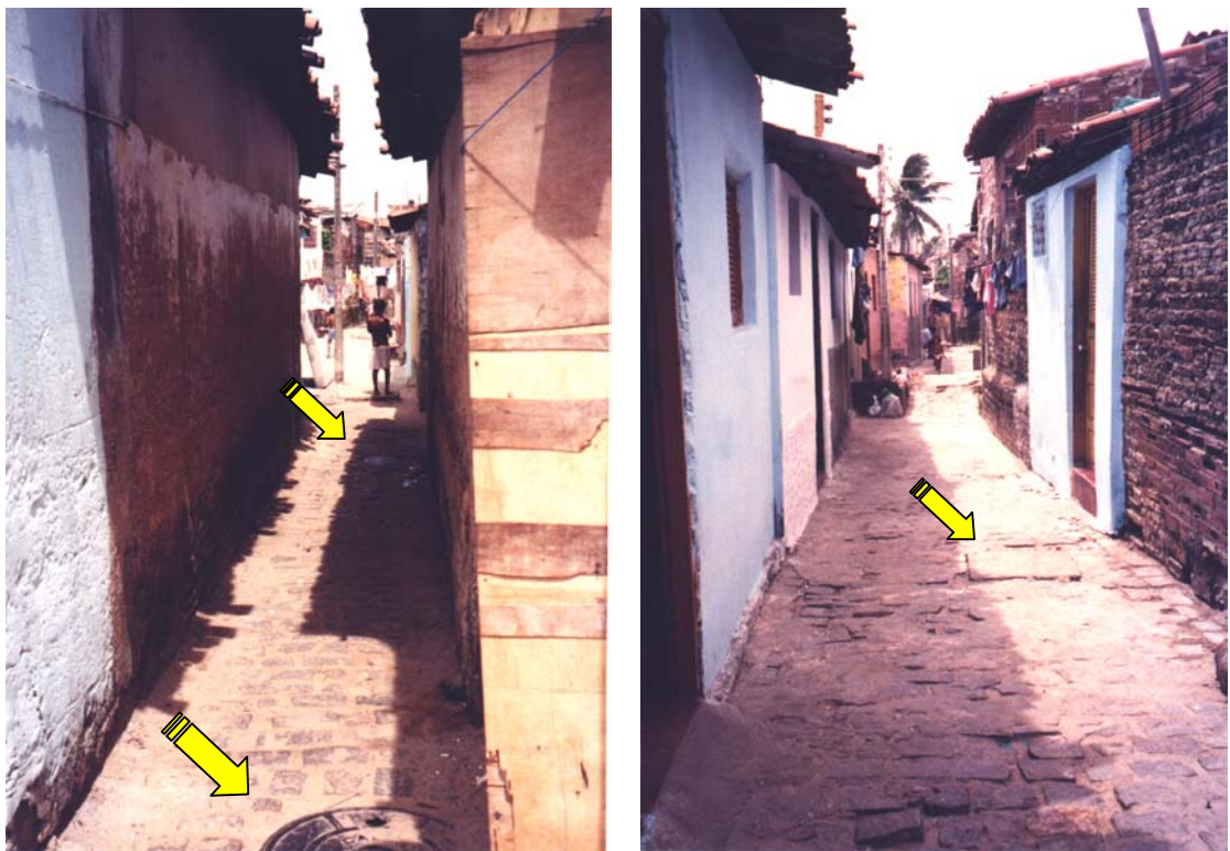
Plate 4.32. Two further views of the Rocas/Santos Reis area, showing condominial sewerage inspection chambers
