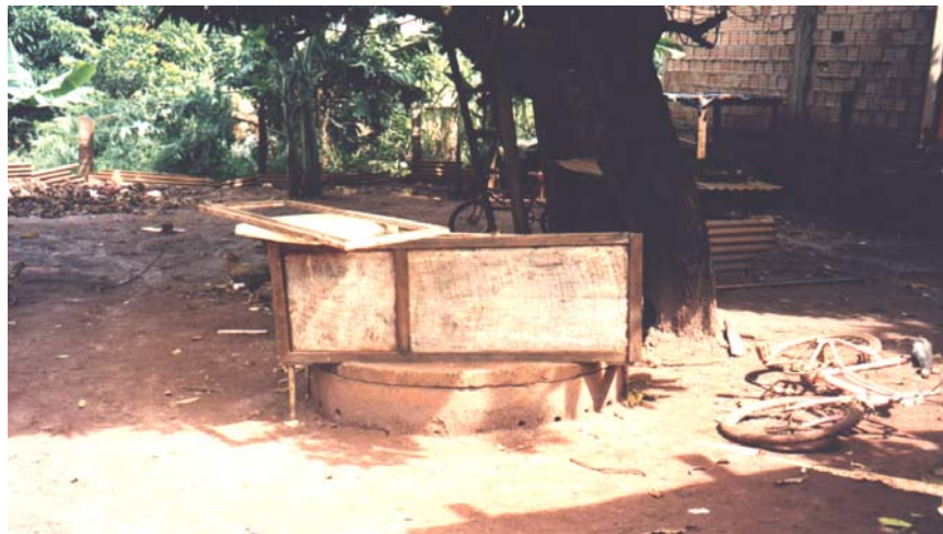
Plate 4.29. Leach pit with exposed leach holes
