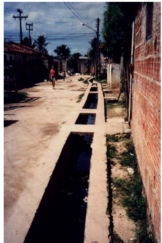
Plate 4.55. Drainage channel in the favela of Poco da Mangueira.
