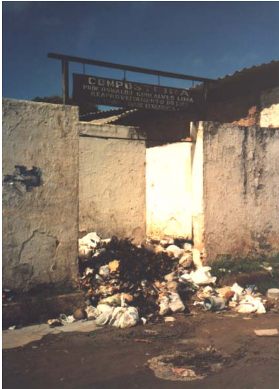
Plate 4.7. The entrance of the composting unit
