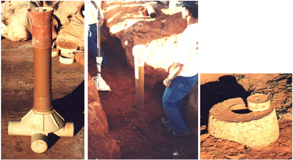
Plate 4.40. In sequence, the condominial TIL unit; soil compaction during the network implementation phase; and the anchorage (protection) of the upper part of the TIL unit.
