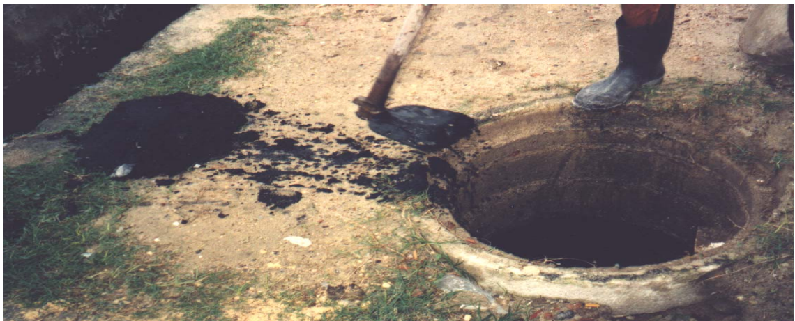
Plate 4.62. Removal of sand from the inspection chamber
