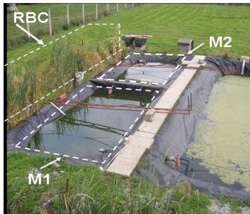
(b) Maturation ponds and reed bed channel
