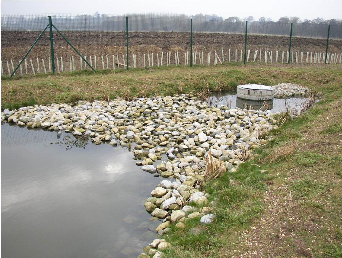
Figure 5.1. Rock filter around the outlet of the facultative pond at Scrayingham, North Yorkshire.
