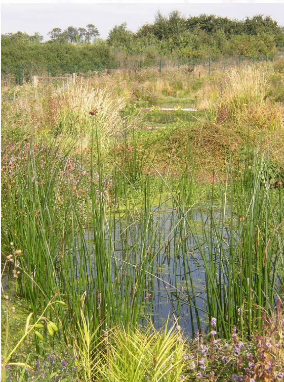
Figure 5.2. Shallow partially planted pond receiving the effluent from the facultative pond at Scrayingham, North Yorkshire, showing the cross-pond gravel filters (top, February 2005; left, August 2005).
