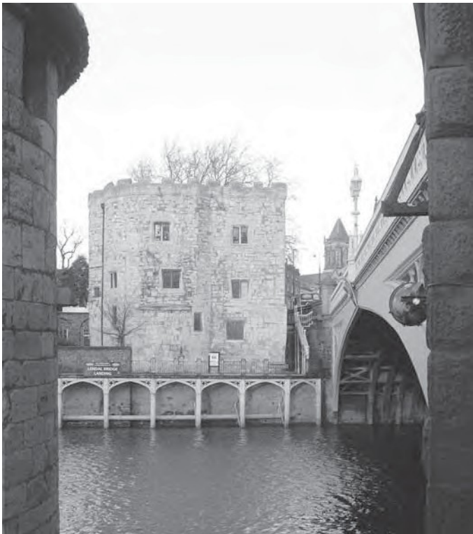
Plate 61. Lendel water tower in Leeds, England, dating back to the 14 th century, in more recent years used as the headquarters of York Waterworks, purchased by Yorkshire Water in 1999 (Photo: Yorkshire Water)
