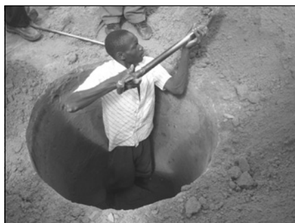
Once the ring beam has been made, the pit can be excavated beneath it.
