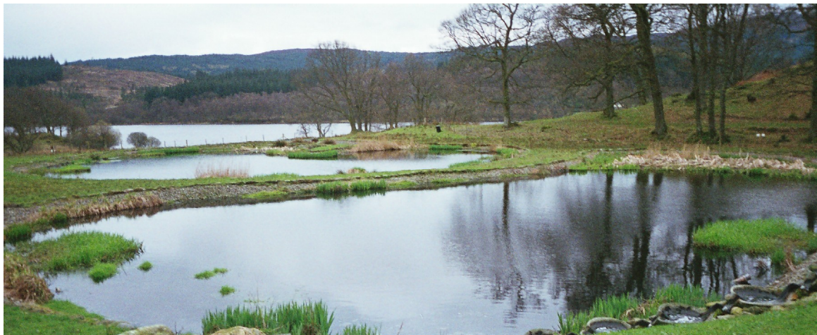
Figure 2. WSP aesthetics: the primary facultative pond at Tigh Mor Trossachs, Perthshire, serving a holiday home complex (top). The facultative pond is followed by two maturation ponds (bottom). The final effluent discharges into Loch Achray (beyond the second maturation pond). Pond design by Iris Water and Design, Castleton, North Yorkshire.
