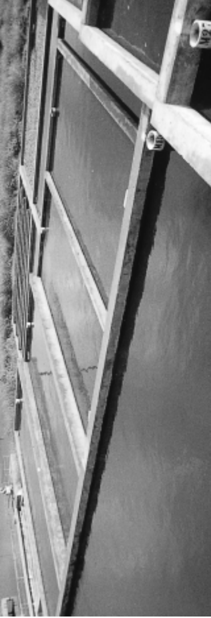
Figure 2.4: Primary maturation (foreground) and secondary maturation ponds at Catingueira.
