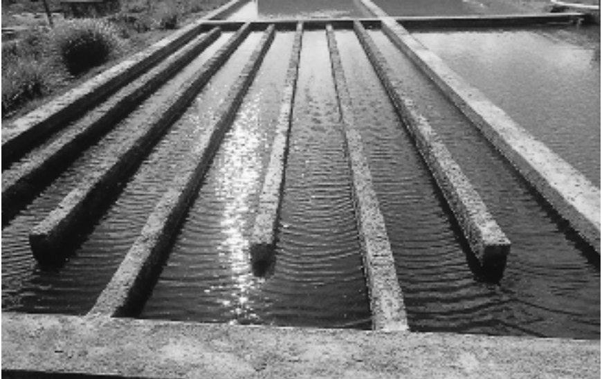
Figure 2.6: Tertiary maturation pond baffled to give a length-to-breadth ratio of 143 to 1.
