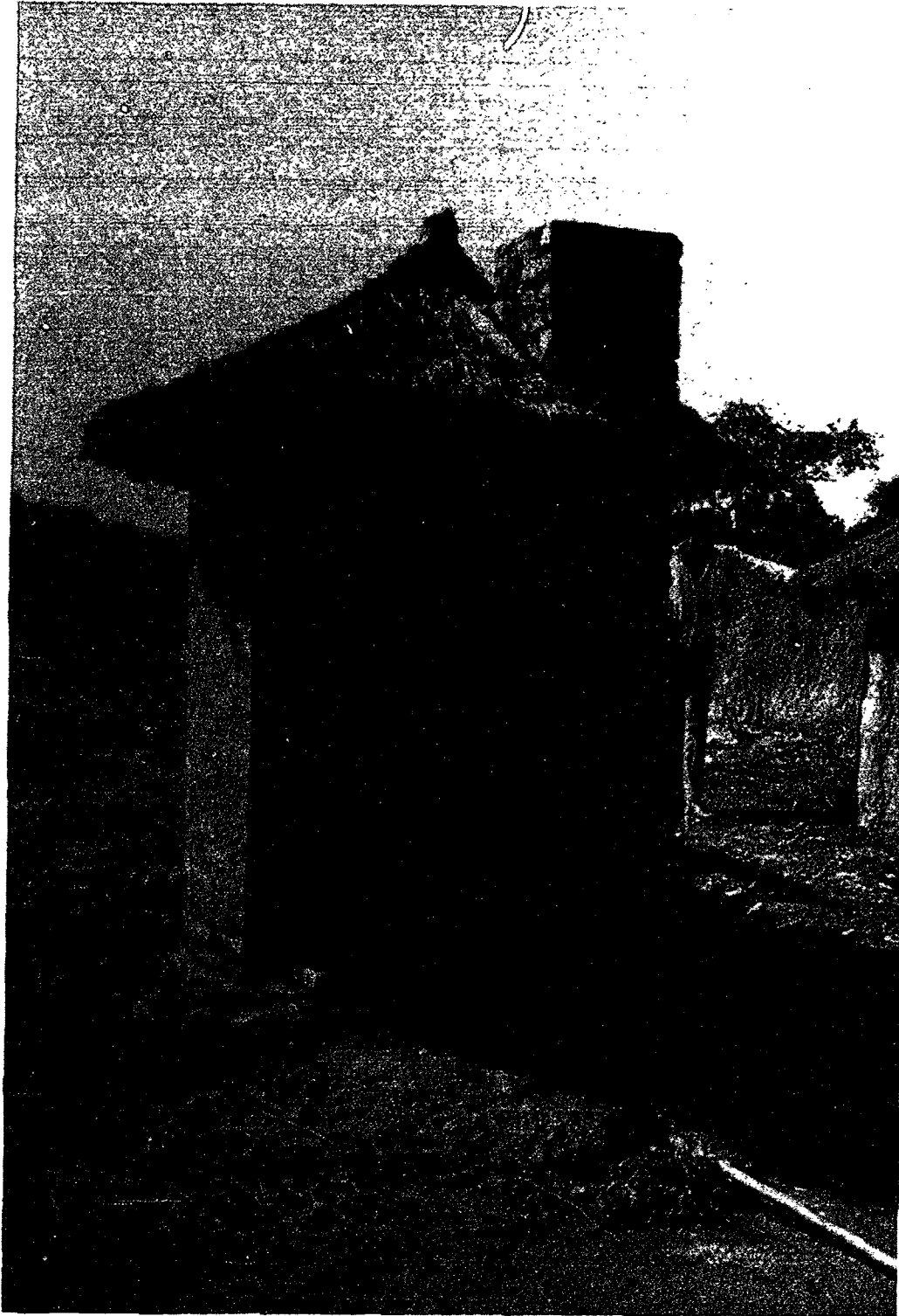
Figure 2. A Blair brick VIP latrine with a brick vent
